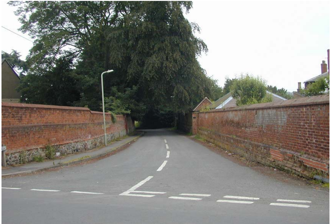
Plate 11 : View South-Westwards along Overton Road from High Street
