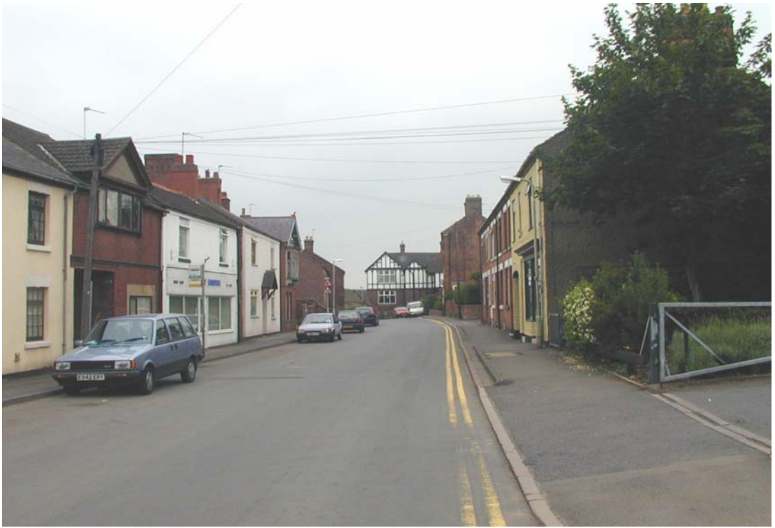
Plate 17 : View South-Westwards along High Street towards Nos. 152/4 High Street
