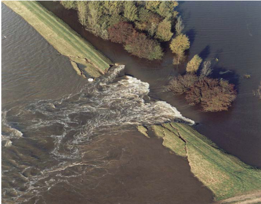
Plate 3 - Breaching of a flood defence embankment (Source: Atkins)
