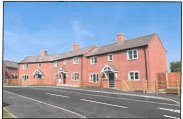
Example of local affordable rural housing scheme at David Taylor Close, Heather
