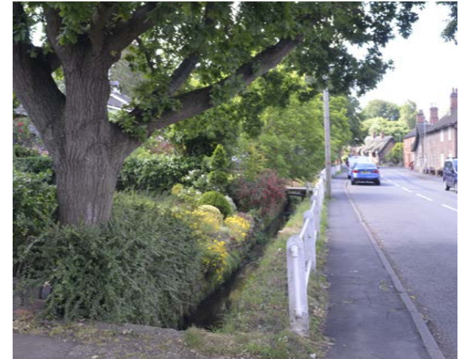
Figure 54: Example of SuDS integrated with a crossing point, Hemington.
