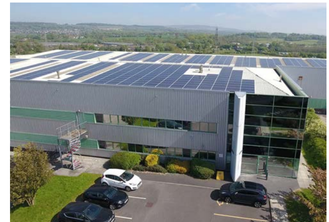
Figure 99: Positive example of large industrial with integrated solar panels on the roof elsewhere
