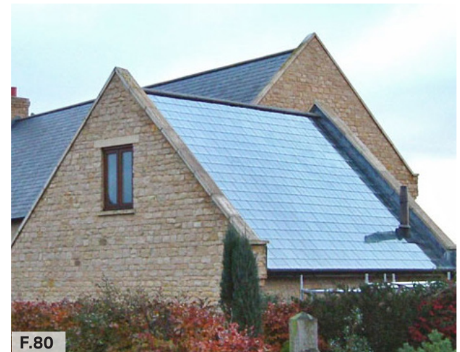
Figure 80: Positive example of integrating solar panels at the design stage.
