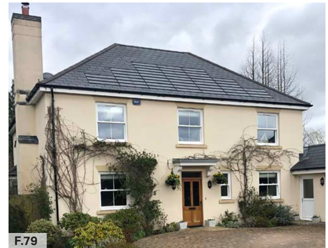
Figure 79: Use of shingle-like solar panels on a slate roof, with the design and colour of the solar panels matching those of the adjacent slate tiles.
