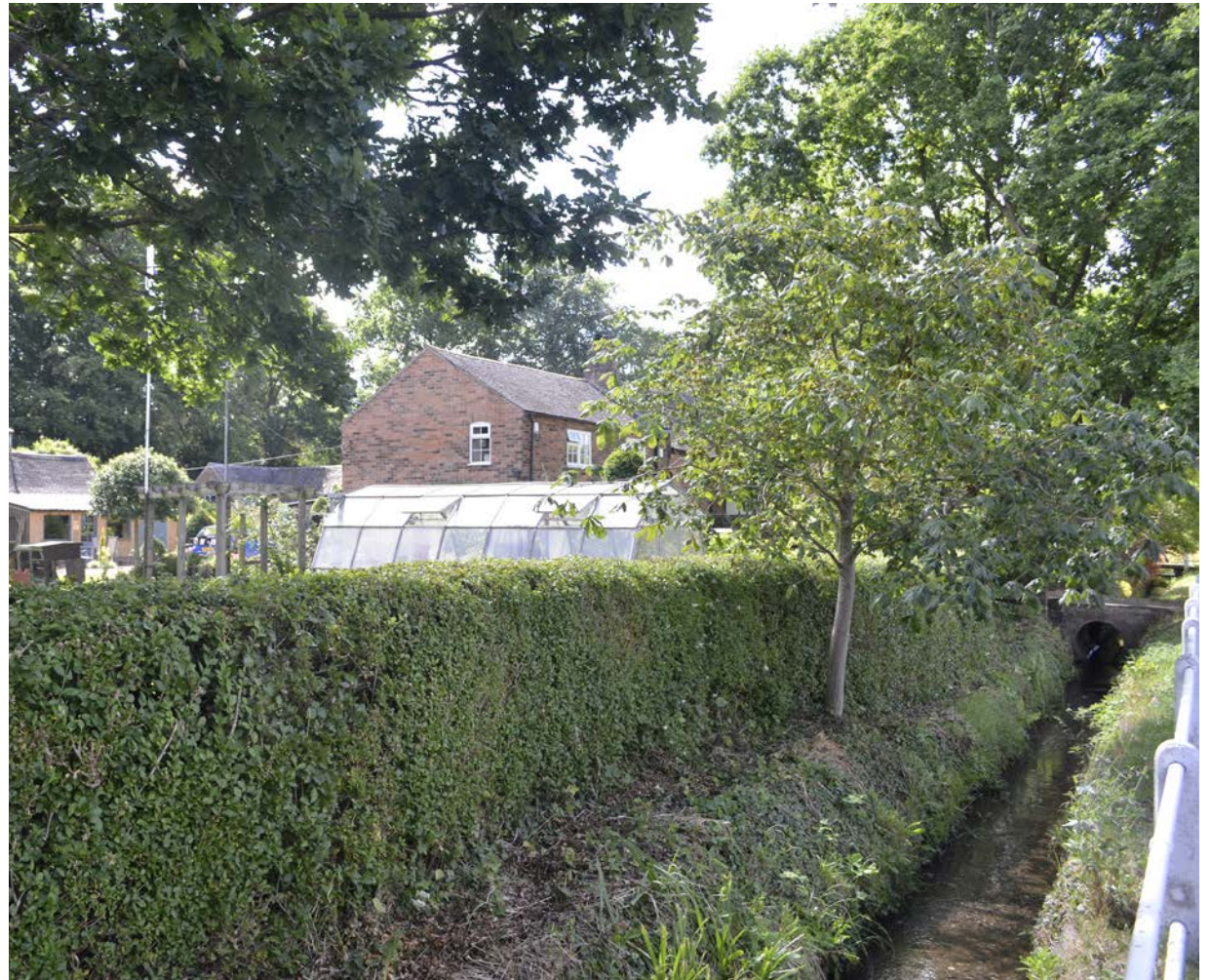
Figure 17: Example of a Sustainable Urban Drainage System (SuDS), in Hemington.
