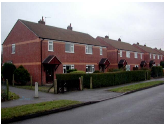
ACHIEVEMENTS: The Council's housing stock is well-maintained
