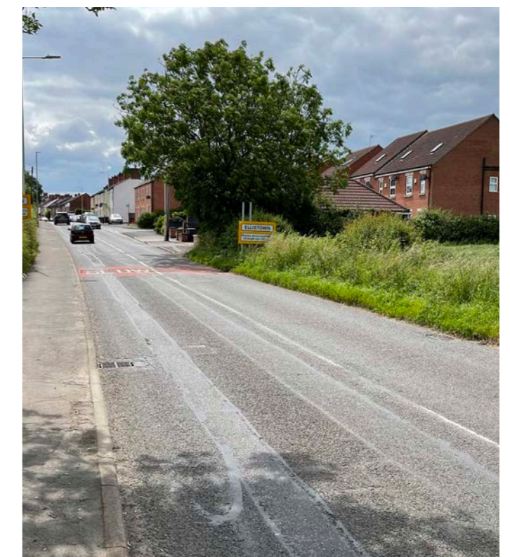
Approach to Ellistown along Midland Road
