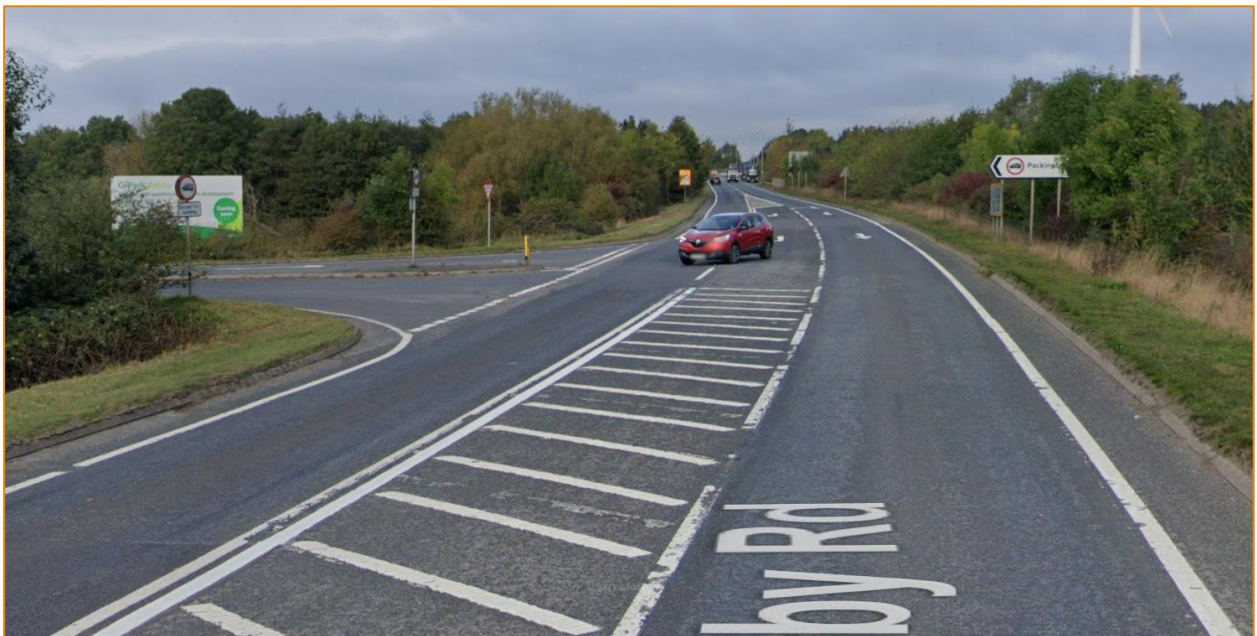
Figure 4: looking northwards along the A511 Ashby Road across its junction with Corkscrew Lane
