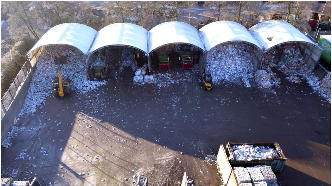
Picture 1 – NWLDC's Waste Transfer Station
