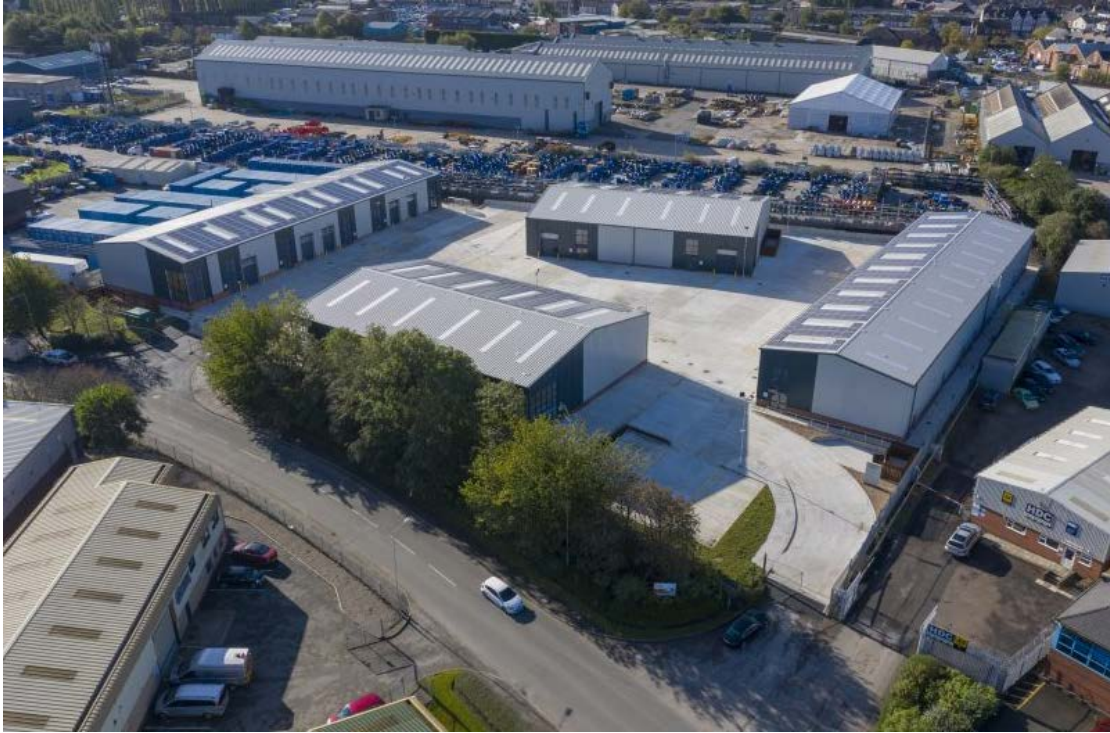
Figure 5-7: Aerial photograph of Apollo Court Business Park
